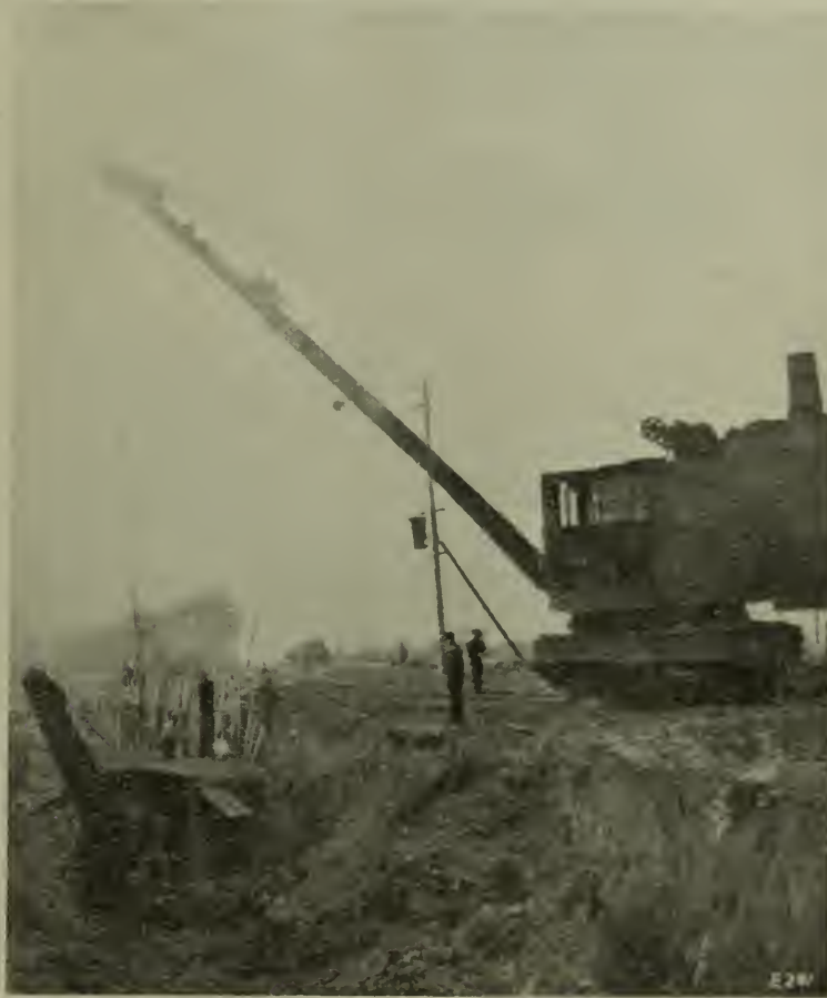
FIG. 4. LOCOMOTIVE CRANE AND GRAB.
